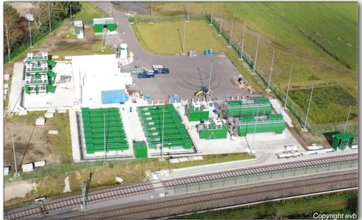
Final refueling station for serial trains
