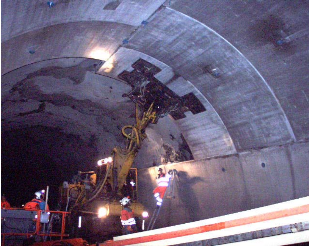
Figur 15: Betong elementhvelv under montering
