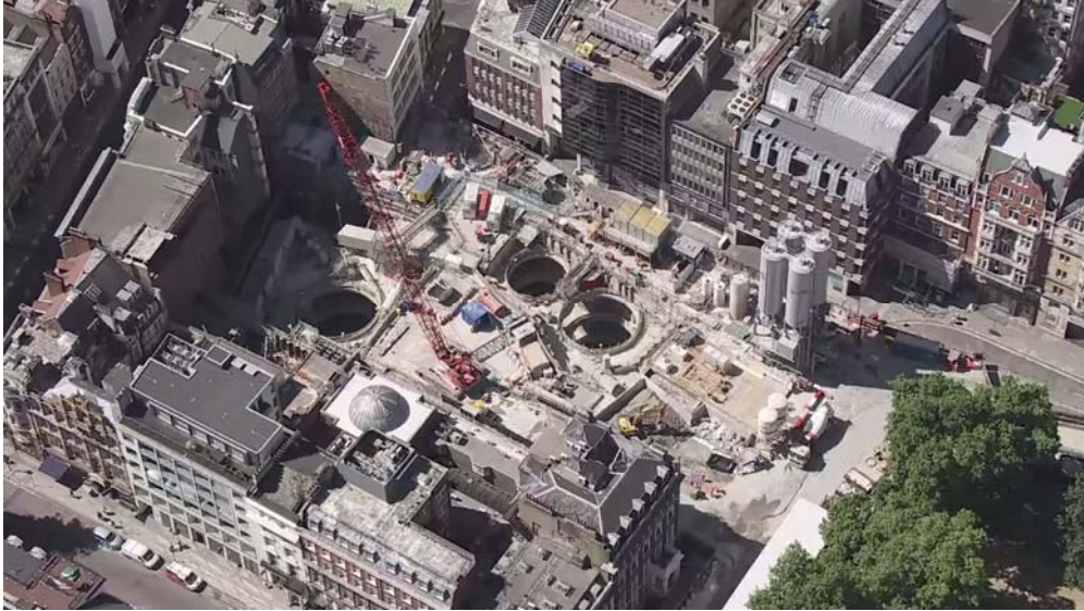
Figure 34: London Crossrail ( http://www.crossrail.co.uk/ )
